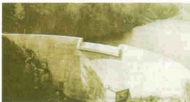
The newly constructed dam as the reservoir fills.
