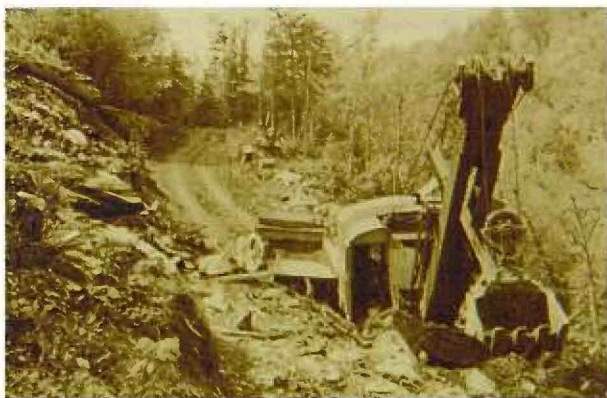
Digging the Dam. One of the first construction tasks was to build a road from Lower Diggin's Road to the dam site, and was started in 1946. The current boat landing and entrance drive to the park were once part of Lower Diggin's road, which is now cut in two by the reservoir.
